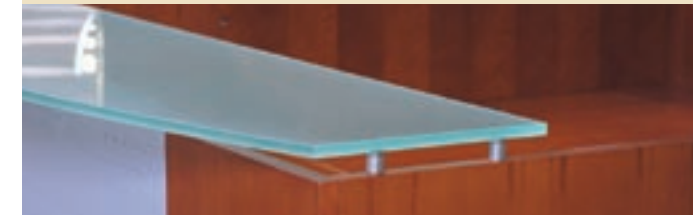
FROSTED 3/4" GLASS TRANSACTION COUNTERS ARE SUPPORTED BY BRUSHED STAINLESS STEEL SUPPORTS.
